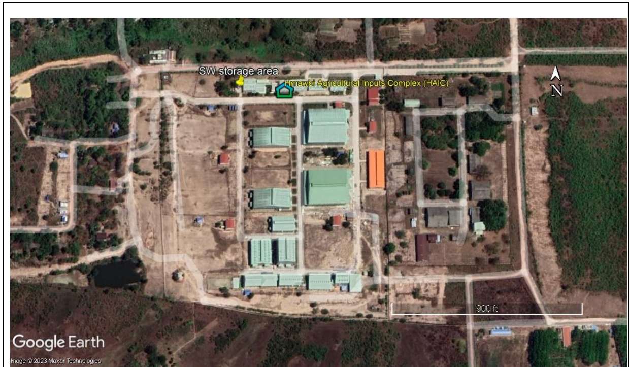
Figure 8-12 Solid waste storage area of Hmawbi Agricultural Inputs Complex
