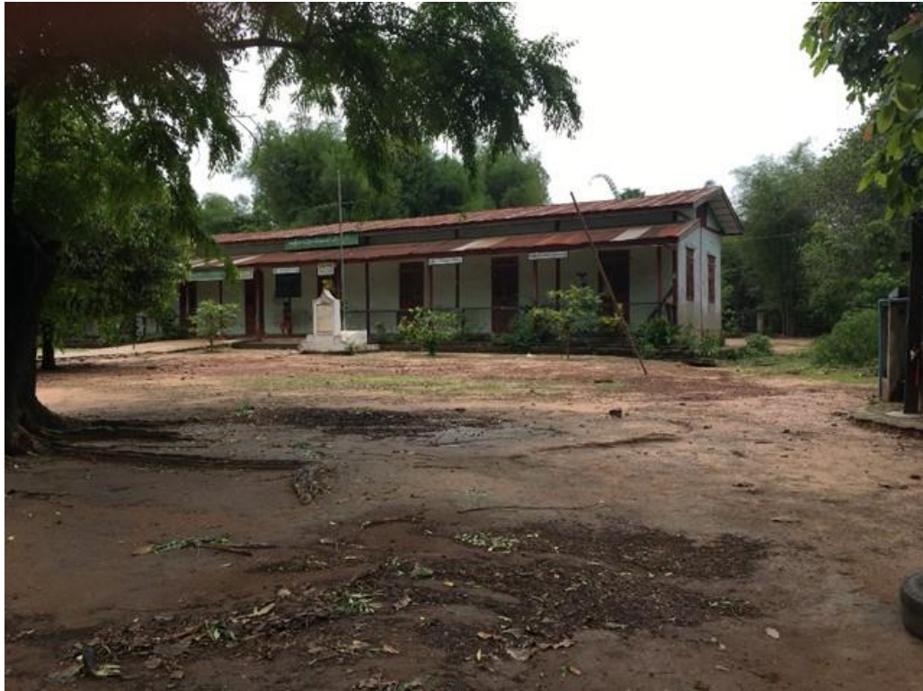
Figure 5.48 Photo Taken from Yae Tar Shey Village
